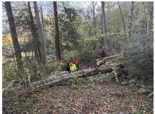
We cleared about 30-35 trees blocking this driveway. Arlin Phillips, Bob Dockery
