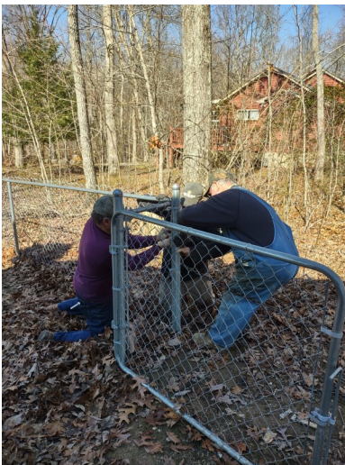
Stretching the fence back in place.
